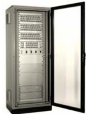
Cabinet for installation of racks
